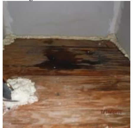
A/C Condensing into Plenum
