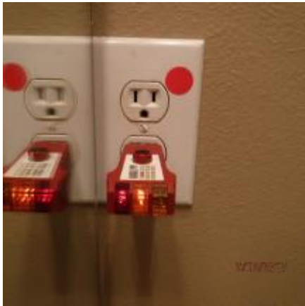
Bathroom Outlet Reversed Polarity
